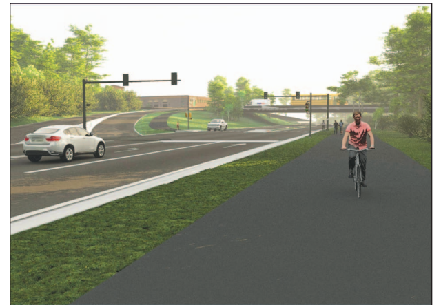
An artist's rendering of the recently approved redesign of Ayd Mill Road with three lanes of traffic (one northbound and two southbound) and a 12-foot-wide trail for bicyclists and pedestrians, looking north toward the ramps to Grand Avenue.
