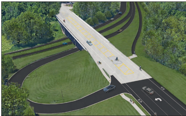
The planned Jefferson Avenue interchange at Ayd Mill Road's south end, with all cars entering Ayd Mill by the ramp on Jefferson's south side and bicycles and pedestrians using the ramp on the north side.
