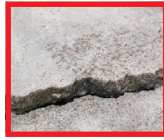
Cracked Concrete
