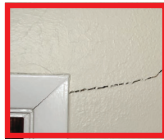
Cracked Drywall
