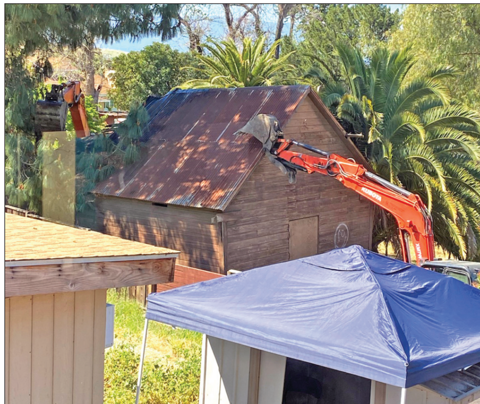
The beginning of the destruction of the old barn.
