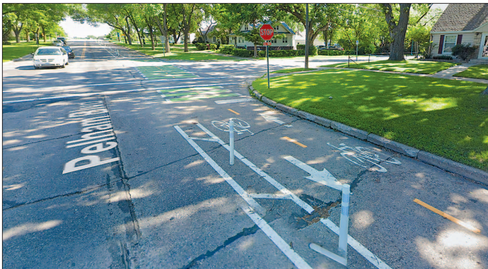
The two-way, separated Pelham Boulevard bikeway was the first of its kind in St. Paul when it was approved in 2017. It also was the first to use white poles to separate bicyclists from motor vehicles.
