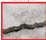
Cracked Concrete
