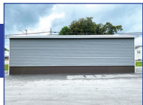
Colonial Beaded Vinyl Siding, Painted Corrugated Metal
