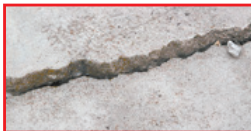
Cracked, Uneven Concrete
