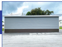
Colonial Beaded Vinyl Siding, Painted Corrugated Metal
