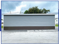
Colonial Beaded Vinyl Siding, Painted Corrugated Metal
