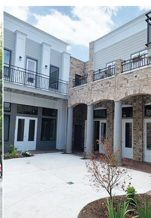
Courtyard view of the “Courtyard”
