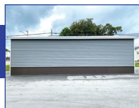
Colonial Beaded Vinyl Siding, Painted Corrugated Metal
