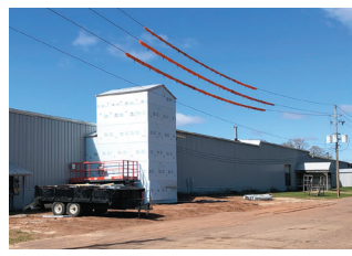
Now complete, GPI started construction earlier this year on a new freight elevator in their main building.
