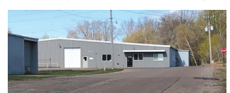
GPI converted a storage building to a production facility.
