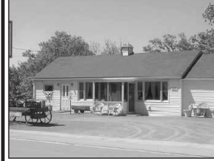
R1198354: NOW $139,900 • ALBION • Presently known as "The Old Goat" - antique shop for the past 6 yrs. • prior to that it was a restaurant for 16 yrs. • 2,188 sq. ft. of usable space (1st floor) • basement semi-finished used as a workshop & storage area • situated on 20.9 acres of wooded land • numerous commercial & retail possibilities • building could be converted to private residence • interior is very charming for any retail endeavor • Call Jim @ 615-0800 for details!
