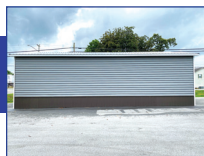
Colonial Beaded Vinyl Siding, Painted Corrugated Metal
