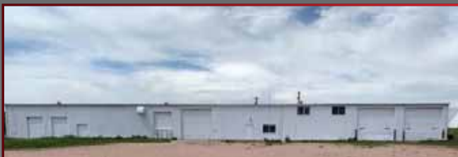
1089 COUNTY ROAD 161 - PINE BLUFFS, WY
