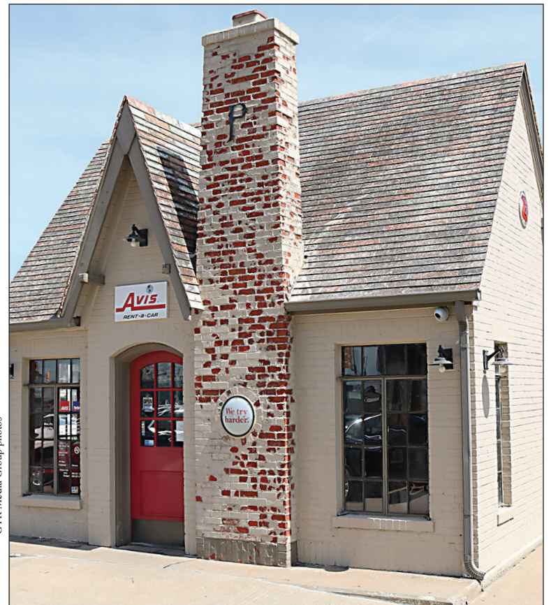
VICKERY PHILLIPS 66 STATION: Located at 602 South Elgin in Tulsa, this former station is listed on the National Register is the home for an Avis Rent-a-Car facility.
