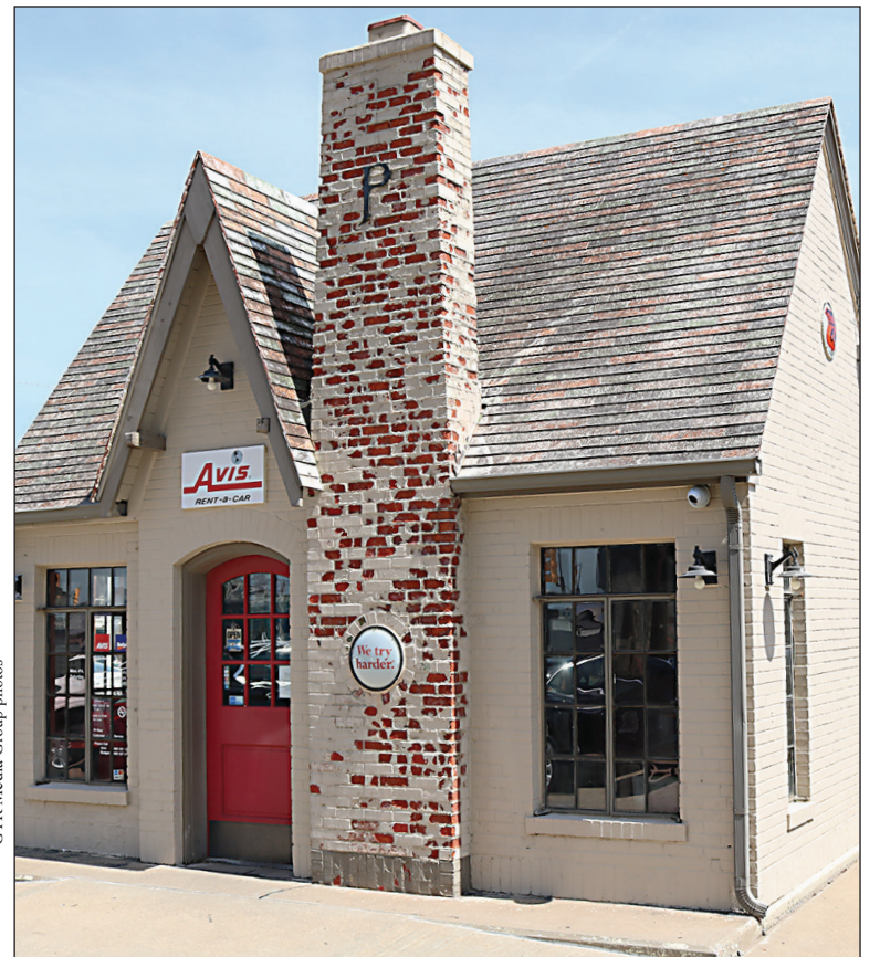
VICKERY PHILLIPS 66 STATION: Located at 602 South Elgin in Tulsa, this former station is listed on the National Register is the home for an Avis Rent-a-Car facility.
