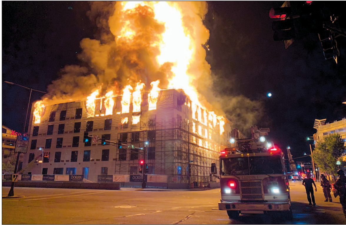
More than 80 firefighters and chief officers responded to control the hotel fire on August 11 at the Seven Corners Gateway site on West Seventh Street in downtown Saint Paul. Crews reportedly were on scene for more than 13 hours. FIRE DEPARTMENT PHOTO
