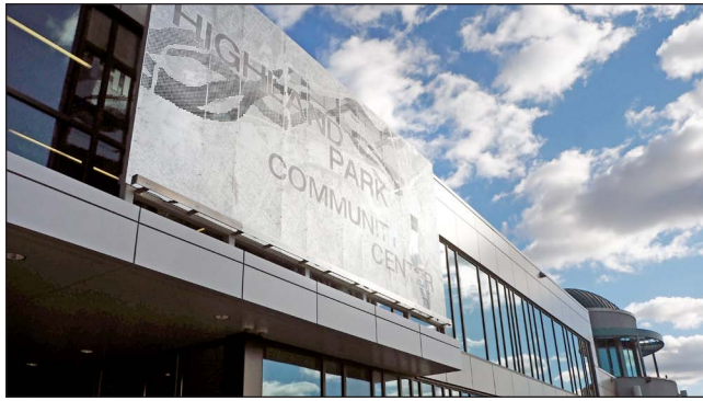
The Highland District Council is seeking CIB funds to redesign the ballfields at the Highland Park Community Center. PHOTO BY BRAD STAUFFER
