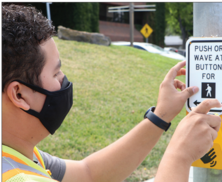
A county worker installs one of the first touchless sensors outside of Valley Med. (Photo courtesy of Santa Clara County)
