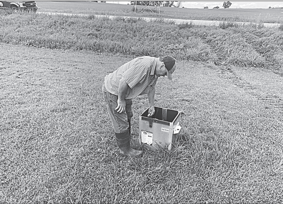
Work is being done to install a filter to help keep phosphorus out of Elkhart Lake.
