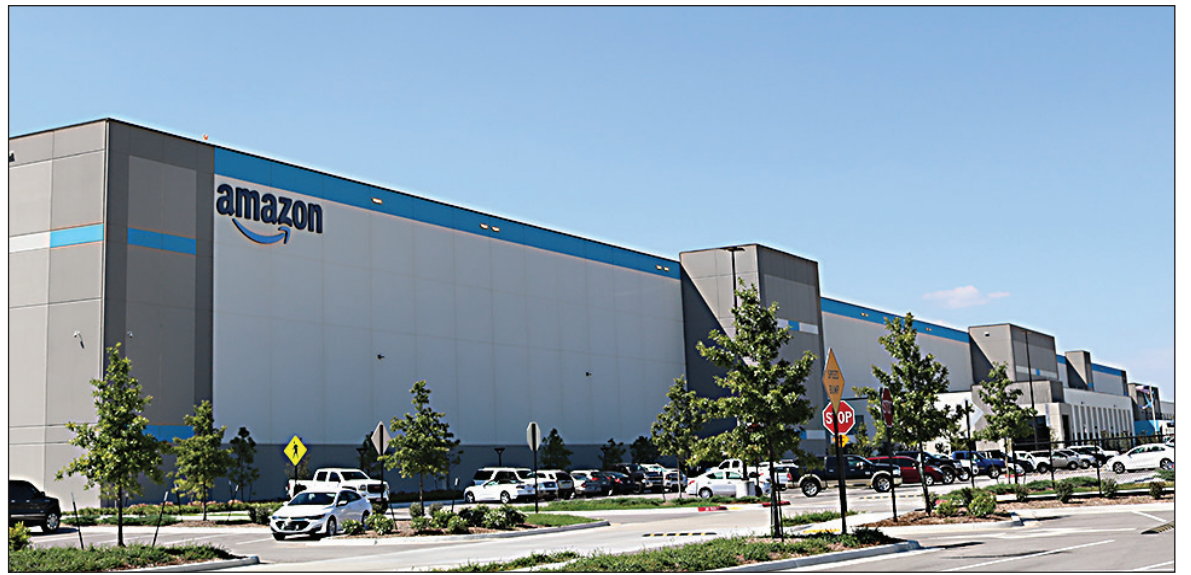
IMPRESSIVE FACILITY: The Amazon 600,000 square-foot Tulsa fulfillment center at 4040 N. 125th E Ave. is a positive economic bonus for greater Tulsa.
