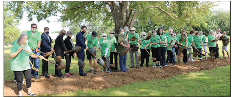
GROUNDBREAKING: Tulsa area officials and future residents break ground for the Heartwood Commons project.
