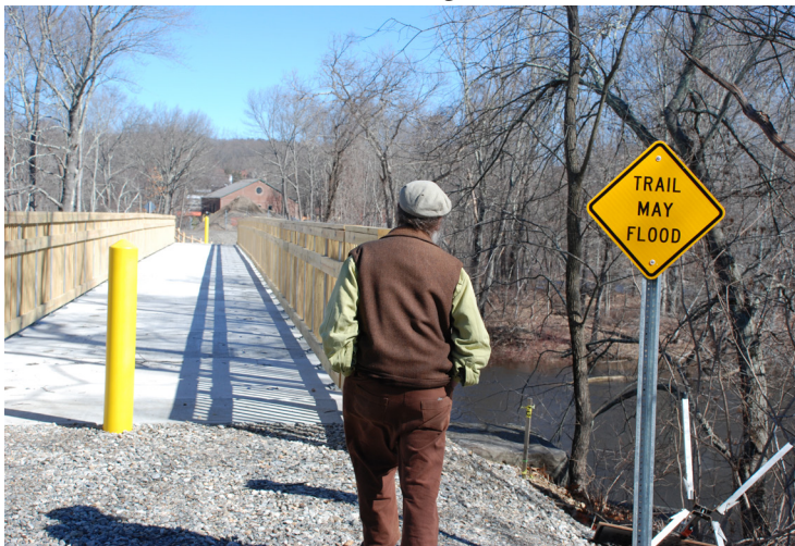
Walking from Lebanon to Willimantic, across the Willimantic River on the new bridge, part of the Air Line Trail State Park. The Railroad Museum is in the distance. Sarah Winter Photo
