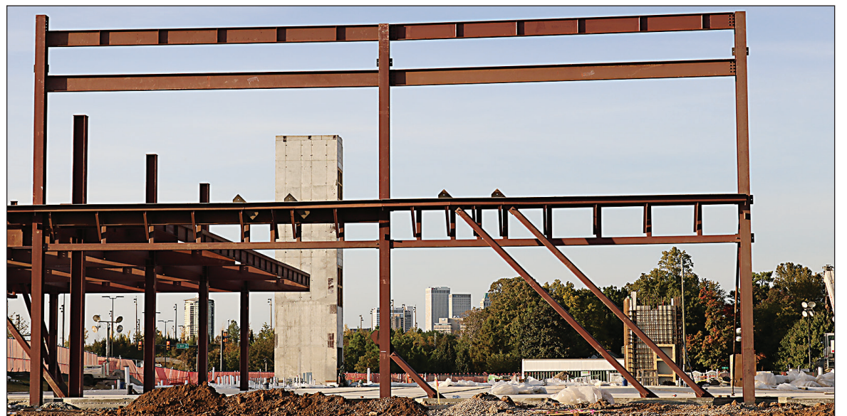
GOING UP: Construction of the Discovery Lab at Tulsa's Gathering Place is progressing for the scheduled opening in the fall of 2021. This photo was taken in early October as construction was beginning. The facility is located along Riverside Drive near East 31st Street at the south end of the Gathering Place.
