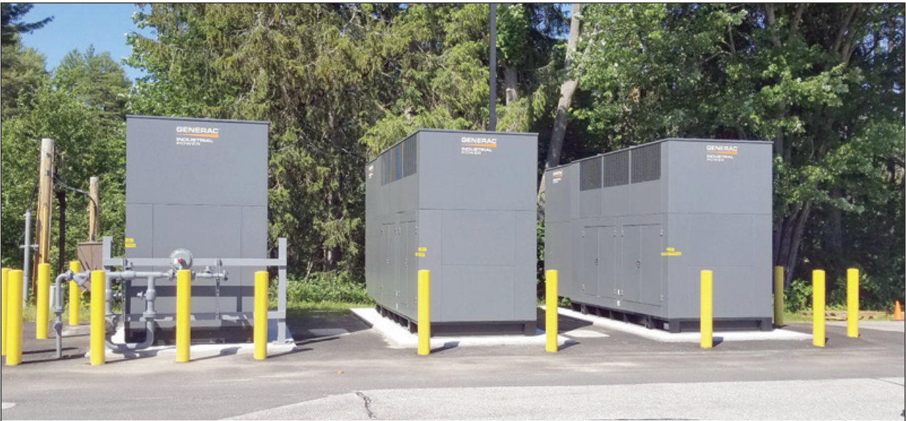
Newly-installed backup generators on the campus of Central Maine Community College enable the facility to become a disaster safety shelter for the local community. (Photo courtesy of CMCC)
