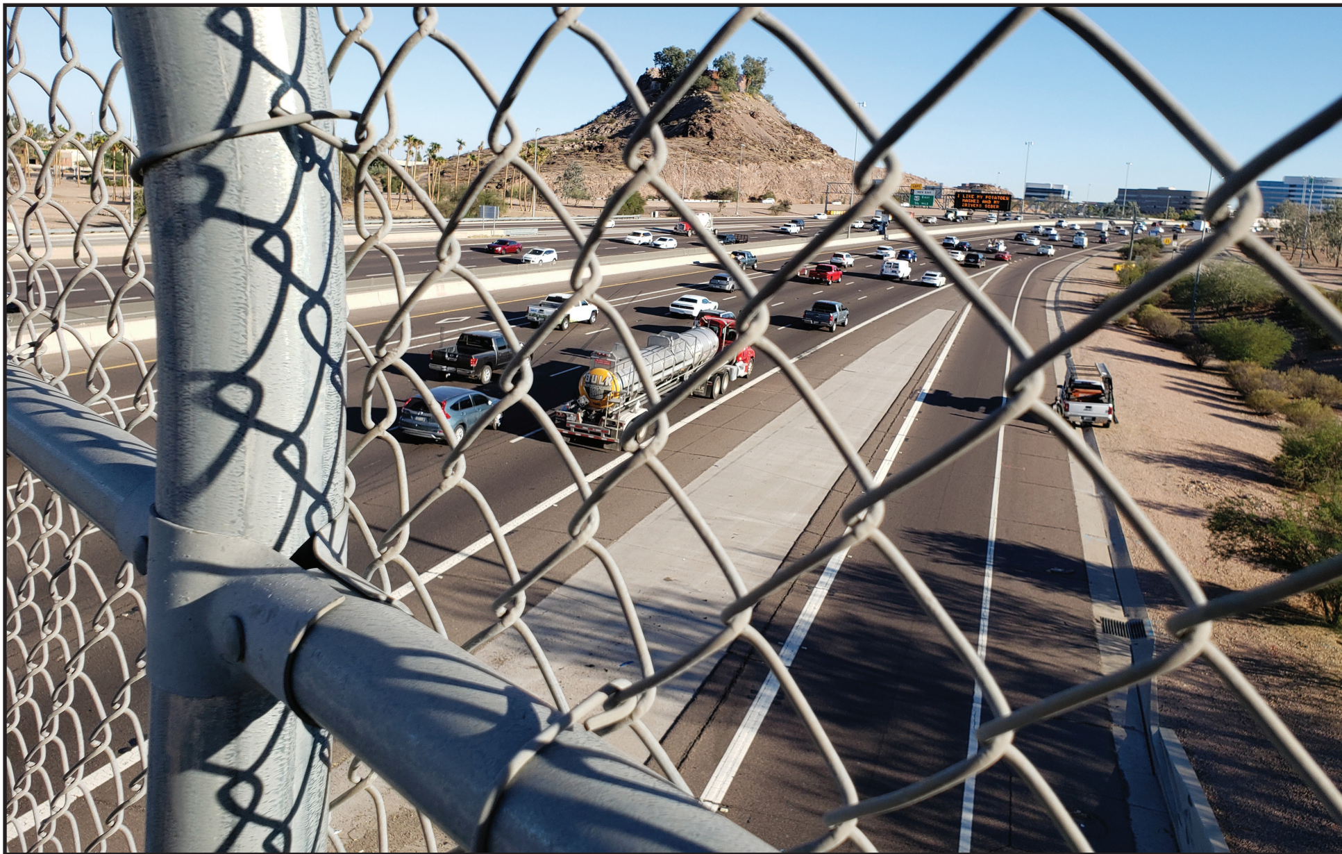
TRAFFIC ON THE BROADWAY CURVE has been a nightmare for years. ADOT is about to fix that.
