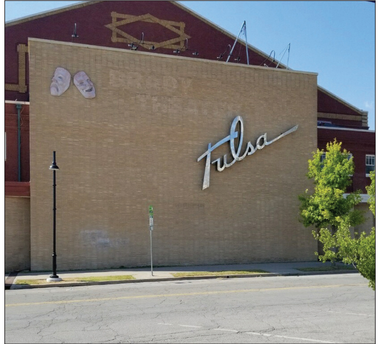
THE TULSA THEATER: The stainless steel sign that adorned the theater from 1952-1979 was resurrected after four decades and recently reinstalled on the buildings north side.
