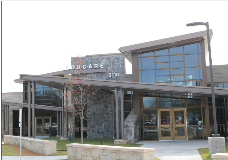
NEW FACILITY: The new Tulsa-based Educare is located around the corner from Celia Clinton School at 3110 E. Seminole St.
