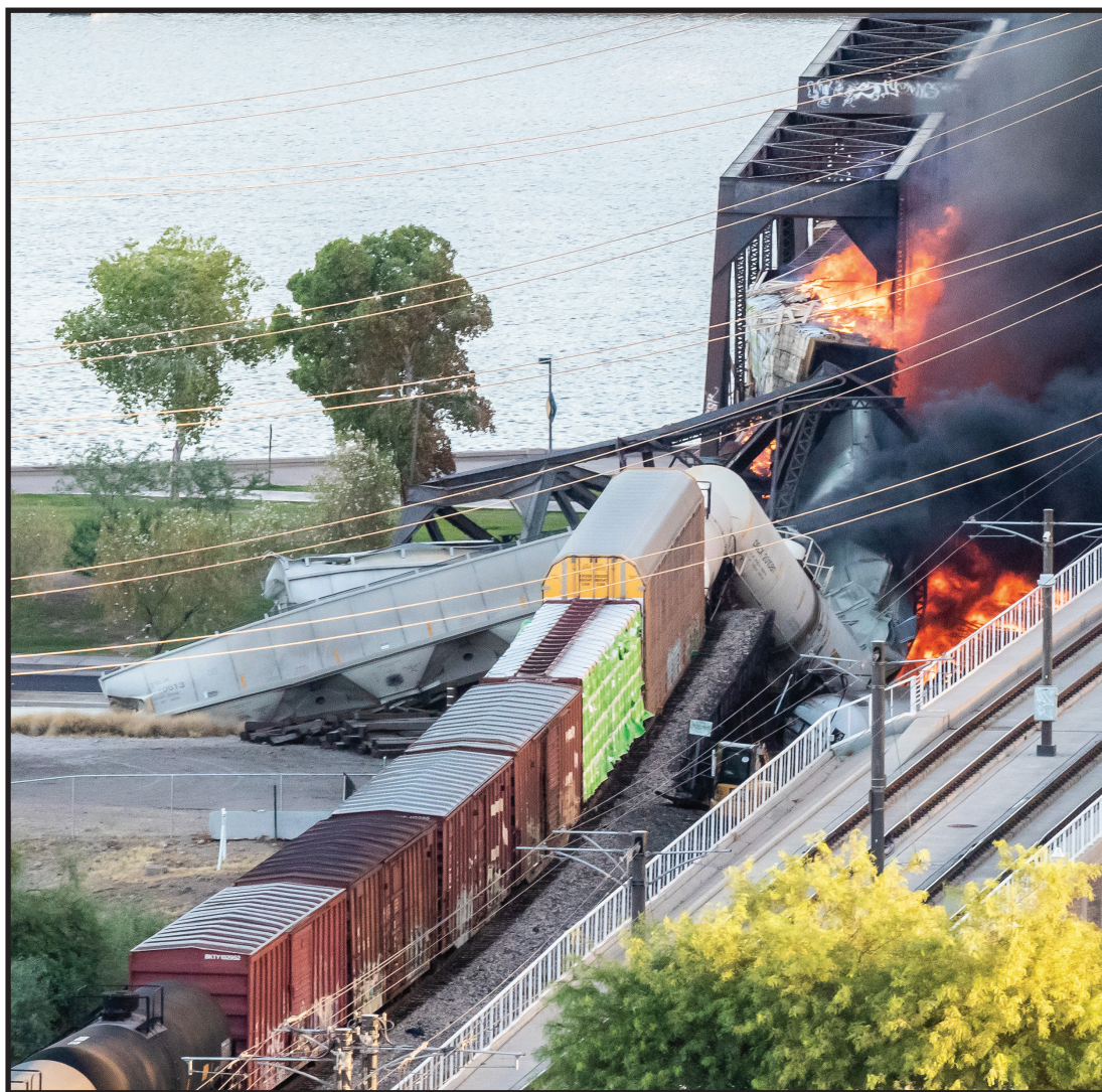
A fiery derailment destroys section of iconic Union Pacific railroad bridge
