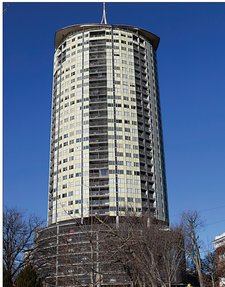
STANDING TALL: Tulsa's University Club Tower building is located at 1722 S. Carson Ave. Built in the mid-1960s, the circular building gives the beautiful Tulsa skyline a unique look.
