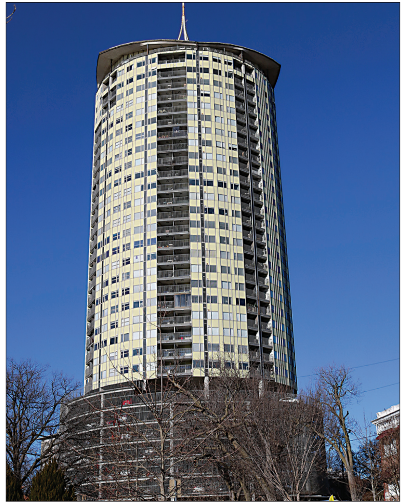
STANDING TALL: Tulsa's University Club Tower building is located at 1722 S. Carson Ave. Built in the mid-1960s, the circular building gives the beautiful Tulsa skyline a unique look.
