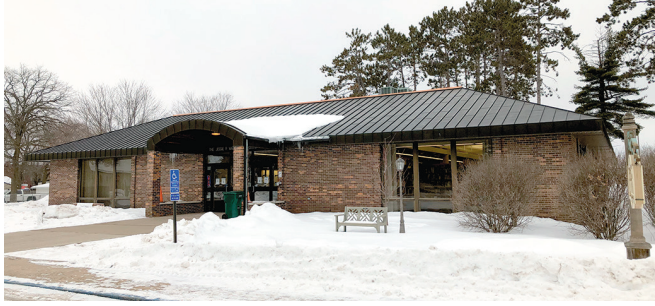
Jessie F. Hallett Memorial Library exterior with new roof.
