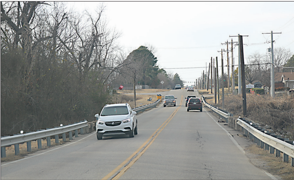
STREET WIDENING UPCOMING: An arterial street widening is coming soon for heavily traveled 81st Street from Memorial Drive to Sheridan Road in Tulsa.
