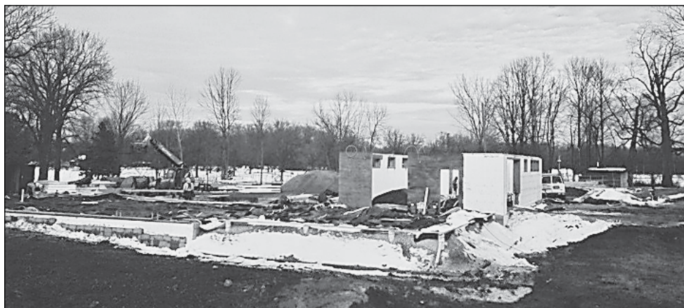
Walls are going up on the Kohler Center for Marsh Education.
