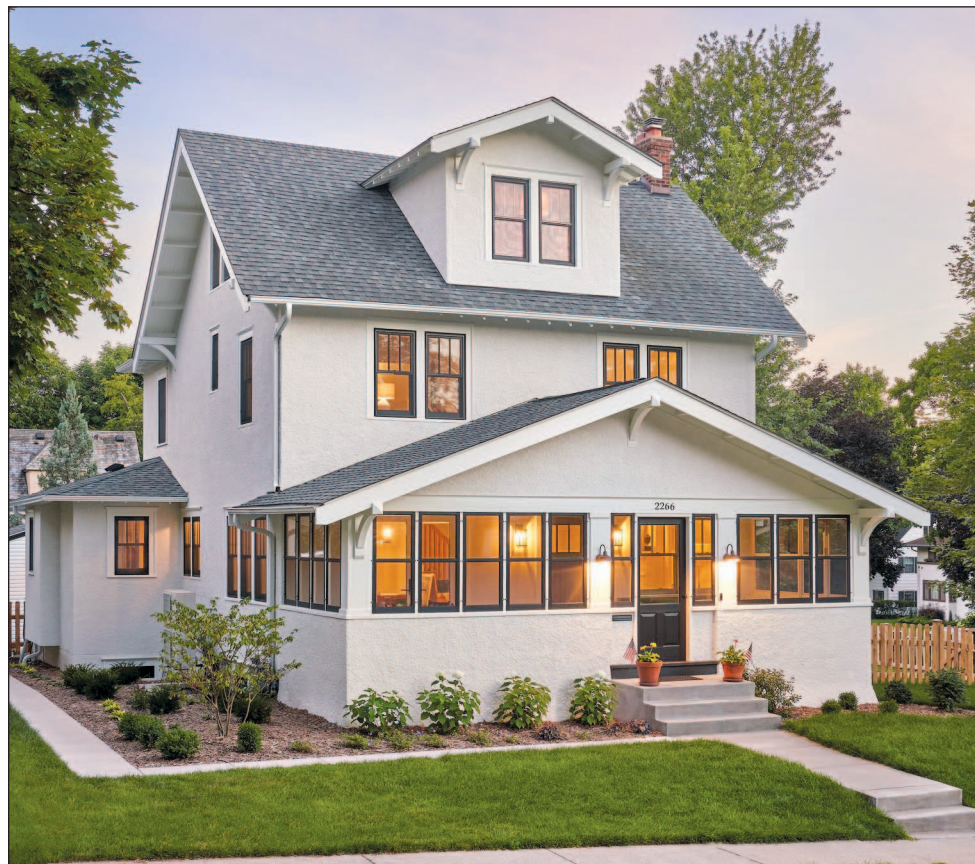
Truly a survivor, this 1917 home is one of 34 that will be open for in-person viewing during the Parade of Homes Spring Remodelers Showcase on March 26-28. PHOTOS BY DREW GRAY
