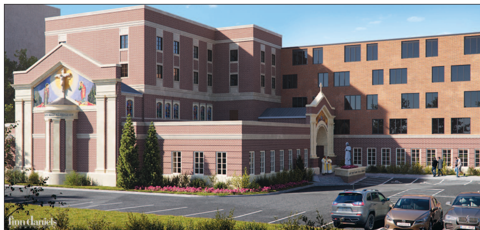
An artist's rendering of the five-story addition to the one-story chapel on the north side of Saint John Vianney Seminary, as viewed from Selby Avenue.
