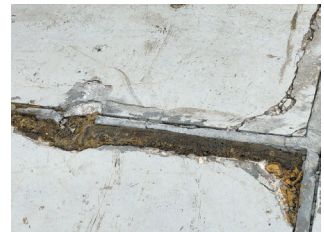
Cracks such as this have developed at the Aitkin Skate Park and need repairs.
