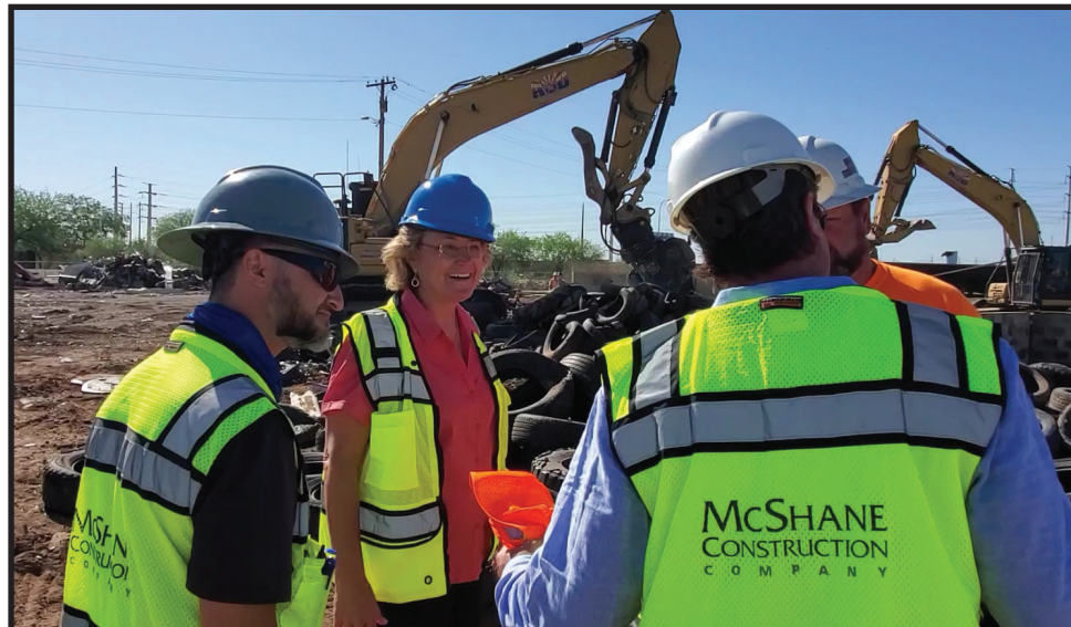
Tempe City Councilmember Jennifer Adams visits the construction site for Banyan North Tempe, an area the city recently annexed. — Photo courtesy Jennifer Adams
