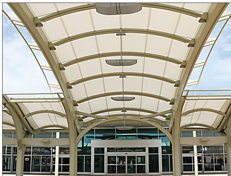
AIRPORT ENTRANCE: The main entrance to the airport is within walking distance from convenient parking.
