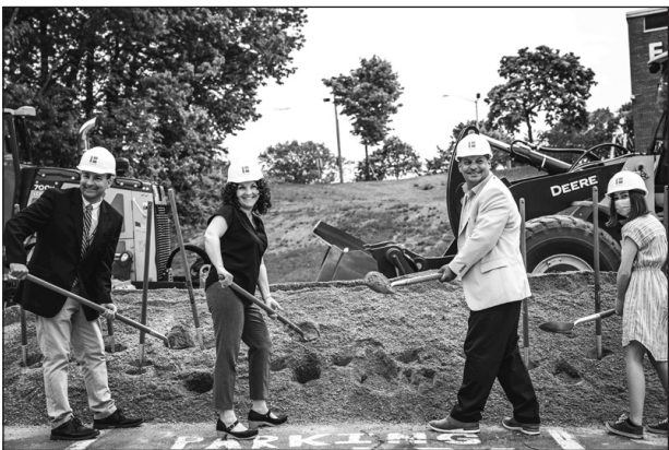
The Auburn School Department broke ground on May 22 for the new Edward Little High School project. (Photo courtesy of City of Auburn)
