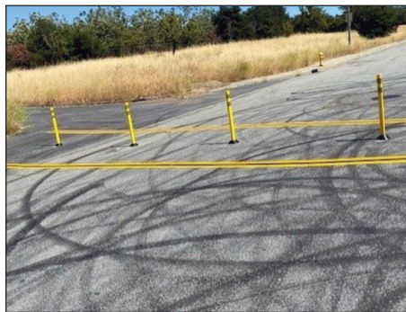
New yellow dividers were added to Yerba Buena Road to discourage sideshows and racing. Courtesy of the city of San Jose.
