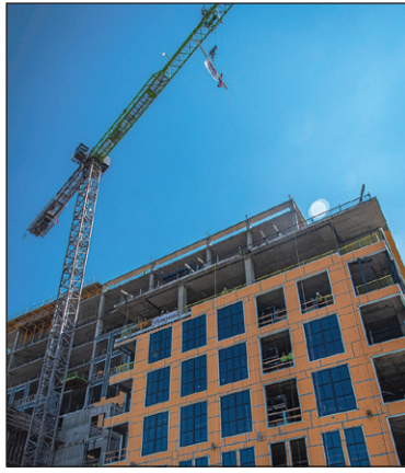
GOING UP: The final beam for the WPX building flies high during the topping out ceremony.
