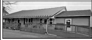
CARLTON – Awesome opportunity with this restaurant/bar! New within a few yrs is the furnace, central A/C, carpeted dining room, industrial kitchen floor, metal roof, patio bar, 10 x 10 walk in freezer & so much more! Screened in patio/bar. Separate bar & dining areas. Seller leaving lots of equipment & supplies. Seller willing to hold the mortgage w/good downpayment & credit. Endless potential!! $199,999 Cheryl Krug Wirth R1106948
