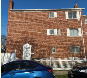
THROGGS NECK LARGE 1 FAMILY BRICK, 3 BED, 1½ BATHS DUPLEX OVER, 1 BED, 1 BATH GUEST SUITE. $698,000
