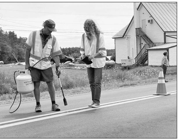
Bicycle Coalition of Maine volunteers heat up a section of the roadway in order to apply mounting plates for traffic delineators on a road in Mount Vernon last Thursday. The delineators help to slow down traffic to improve safety for bicyclists and pedestrians on roadways. (Photo courtesy of BCM)
