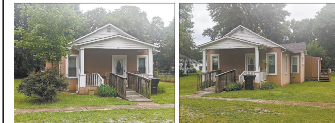
Come bid and buy at your price on this 2 bed / 2 bath home. Property features, nice front porch; roof, siding, HVAC and appliances updated around 2012; 22X 14 deck.
