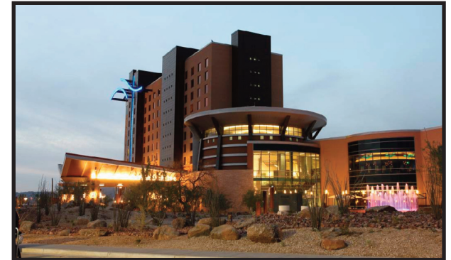
A new tower opens this fall at Wild Horse Pass Hotel and Casino that will nearly double capacity to 447 rooms.
