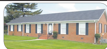
#874 - Well-maintained brick ranch-style home convenient to town. 3BR / 2BA, formal living and dining, eat-in kitchen, family room w/ built-ins, tile baths, 2 car attached garage, concrete drive, nicely landscaped. Seller is the original owner. MLS#1666784 $125,000
