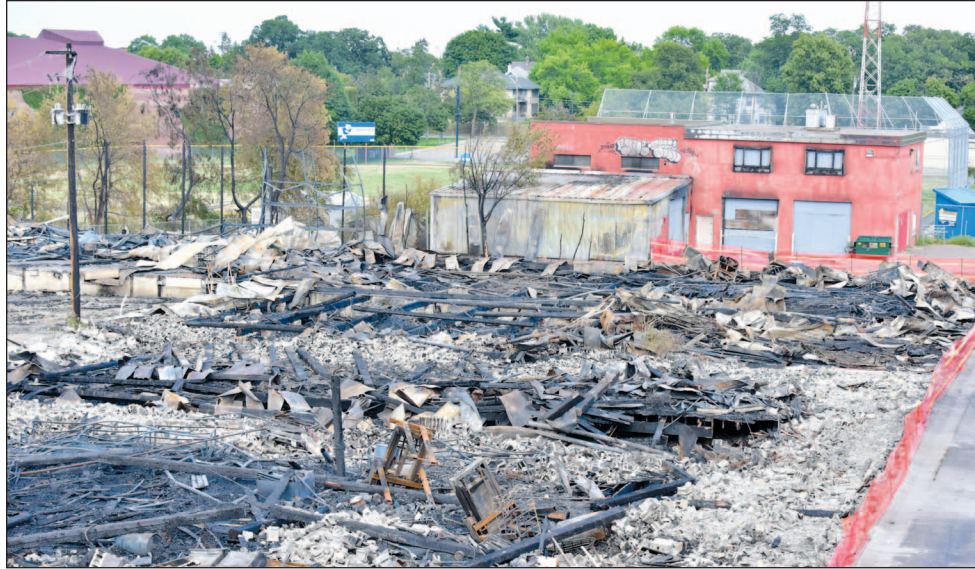
Snelling-Hamline warehouse fire. The aftermath of a three-alarm fire on August 21 that destroyed a warehouse complex at 1400 Dayton Ave., just behind the Concordia University baseball field. The fire was reported at 5:43 p.m. and it took 86 fire personnel more than 21 hours to get it under control. Plumes of black smoke could be seen for miles, due to vehicles, auto parts and tires stored in the four buildings. No injuries were reported. Arson is suspected. PHOTO BY CHAS JENSEN
