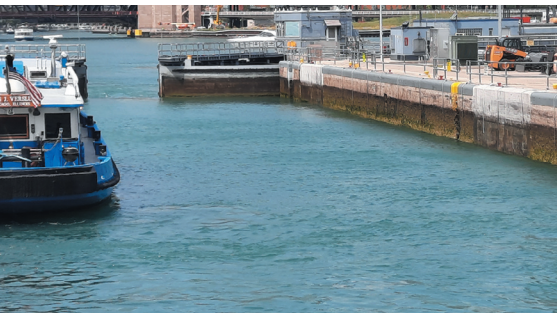
View of the lock at the Chicago River's entrance to Lake Michigan. Note the dark water markings on the side. The river is approximately three feet lower than the lake.
