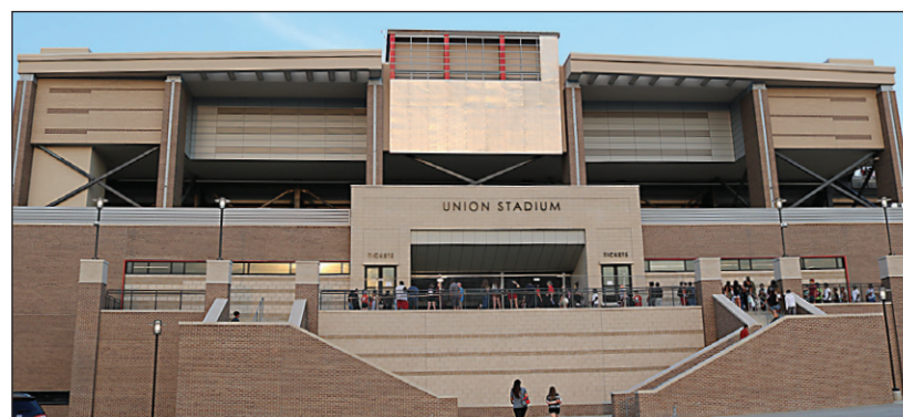
UPGRADED ENTRANCE: The main entranceway to the rebuilt Union Tuttle Stadium is located on the west side near the UMAC (Union Multipurpose Activity Center).
